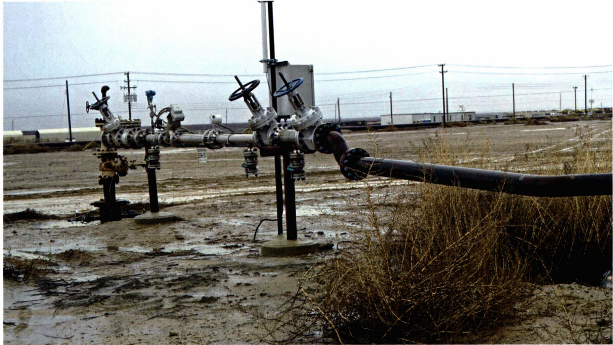
A wastewater injection well in San Joaquin County. (Lauren Sommer/KQED)
