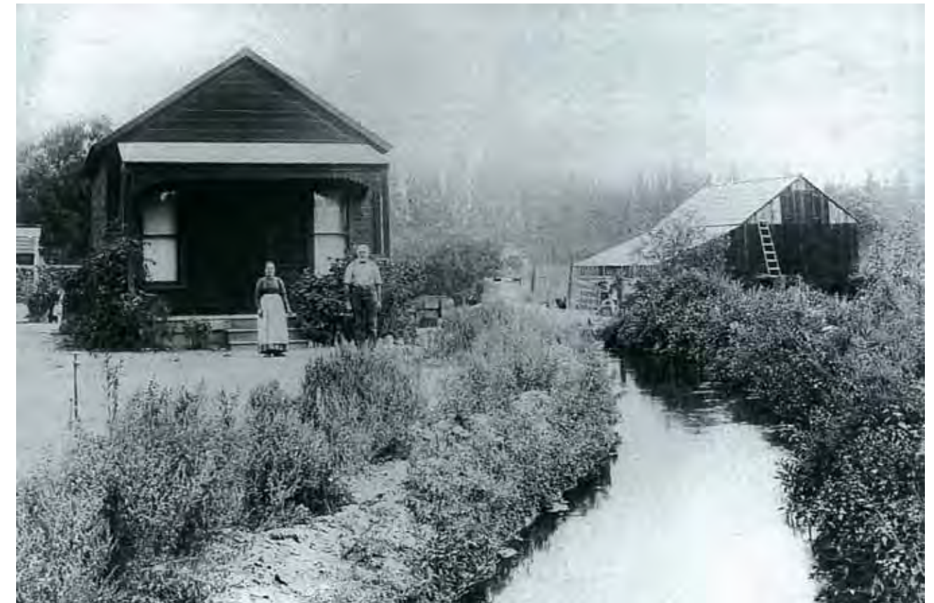
Fig. 2.8. Diversion ditch from Santa Paula Creek, ca. 1900. Surface diversions, such as this ditch taking water from Santa Paula Creek downvalley, brought water from areas with abundant surface flow to drier portions of the valley. (Unknown ca. 1900a, courtesy of the Santa Paula Historical Society)
