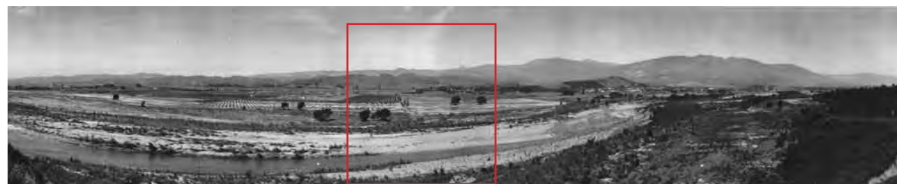
Fig. 3.25. This image of the Santa Clara River west of Santa Paula was taken on March 17, 1928—only five days after the St. Francis Dam break swept through the Santa Clara River valley. The recent presence of high flows is evident in the low vegetation along the river, which is bent downstream in the direction of flow. Even after such a large event, riparian patterns are evident: live oaks are seen bordering the river, while the bottomland surfaces are dominated by low scrub. The active channel is largely unvegetated, having been recently scoured by the flood. (Isensee 1928b, courtesy of the Museum of Ventura County)
