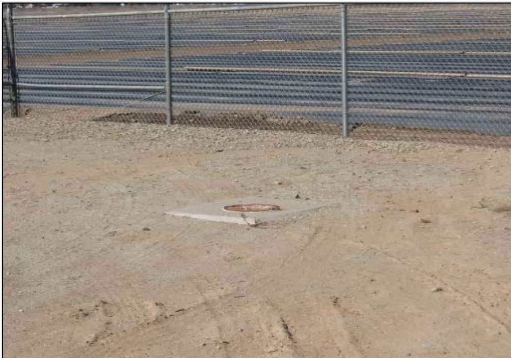
Figure 3: Completed monitoring well with flush pad and vault.
