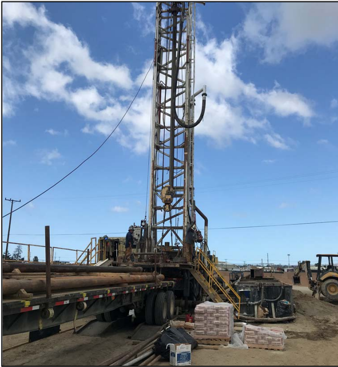
Figure 6. Reverse-rotary drill rig.
