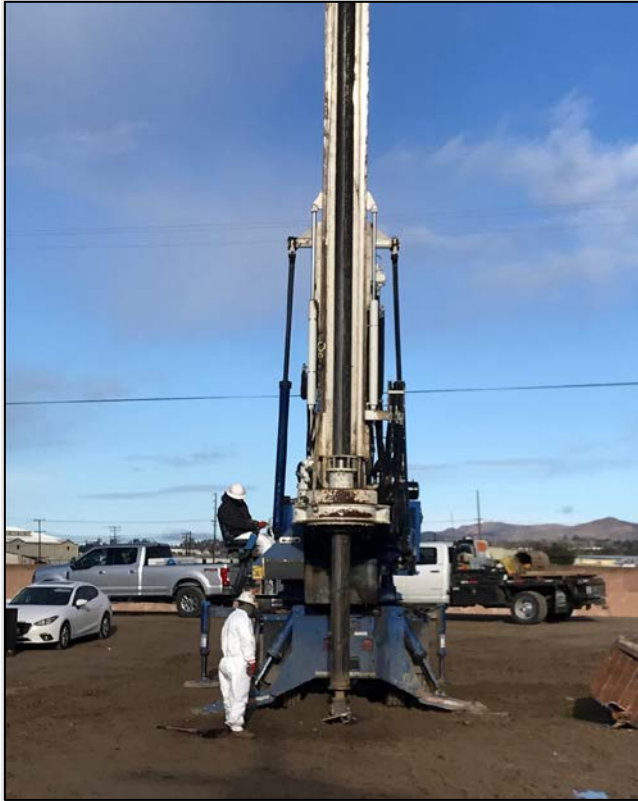
Figure 4: Example auger drill rig.
